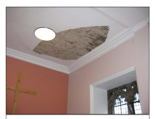
Visitors to Holy Trinity over the past few weeks will have noticed the hole that has appeared in the ceiling in the Vestibule. This is apparently due to some water damage to the plaster which caused it to come away from the lathes. The root cause is thought to be a leak in the zinc roofing above the area.
